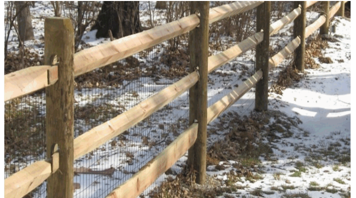
Split Rail with wire mesh
