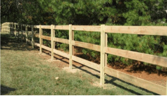
Kentucky Board without wire mesh
